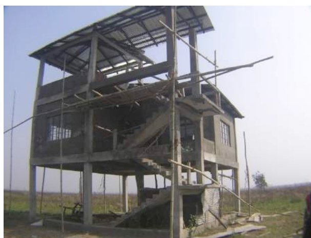
Figure 2. IRV 2020-funded infrastructure improvement in Manas National Park
